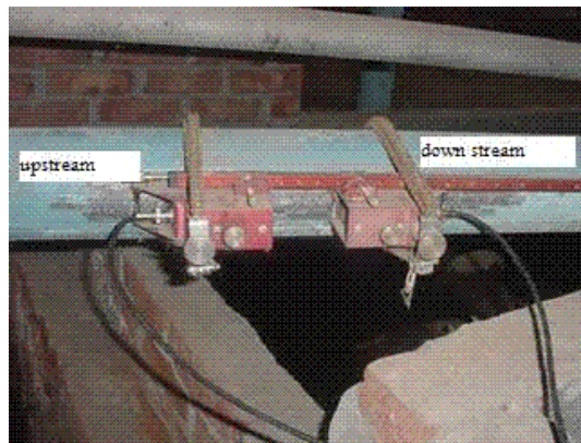
Figure (11): Mounting U-S. flowmeter on steel pipe.
